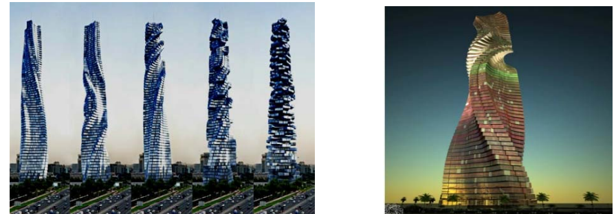
Picture 5 – Da Vinci Tower
