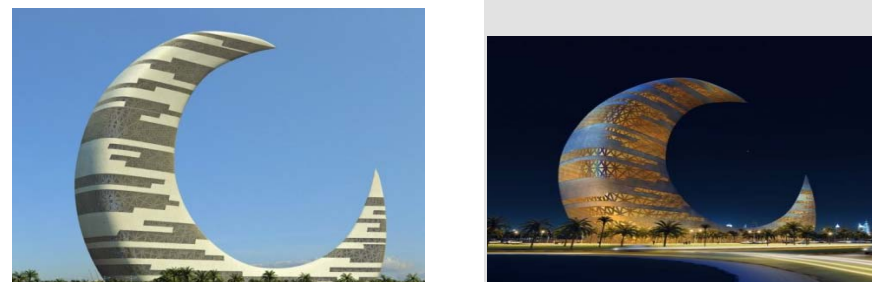
Picture 10 – Crescent moon Tower
