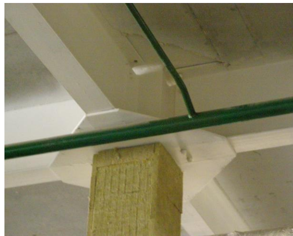
Fig. 2. The joint of the steel beams on the column
