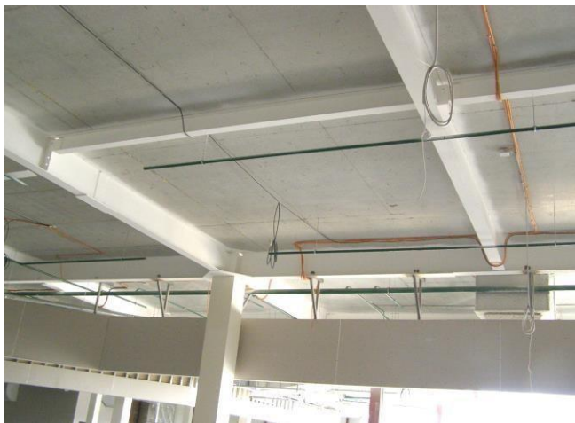
Fig. 1. View of a steel-reinforced concrete floor fragment
